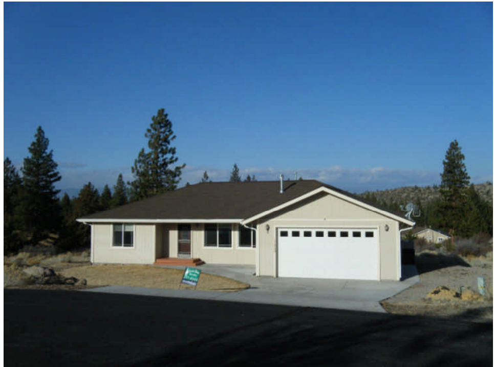
Inspection conducted by, DON HANSEN CCI Certified CREIA Inspector
